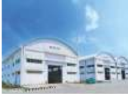
DG Set Manufacturing Unit 1-Kathua, J&K
