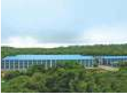
DG Set Manufacturing Unit-Kalsar, Gujarat
